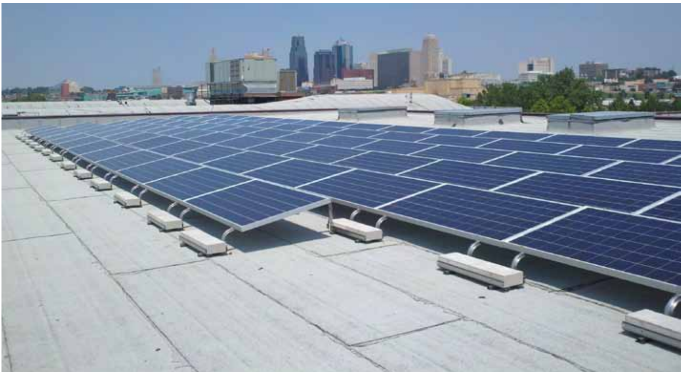
Rooftop solar panels on top of the historic Gem Theater in Kansas City, Missouri.
